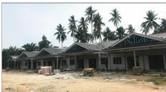
Under construction, Taman Perigi Nenas Kg Perigi Nenas (June 2019)
