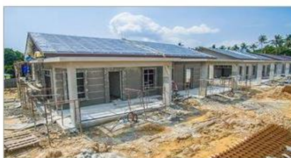
Under construction, Kg Perigi Nenas (December 2019)
