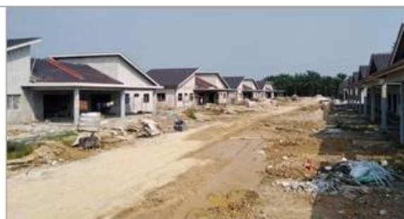
Under construction, Taman Perigi Nenas Kg Perigi Nenas (December 2019)
