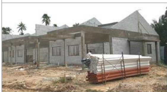
Under construction, Kg Perigi Nenas (December 2019)
